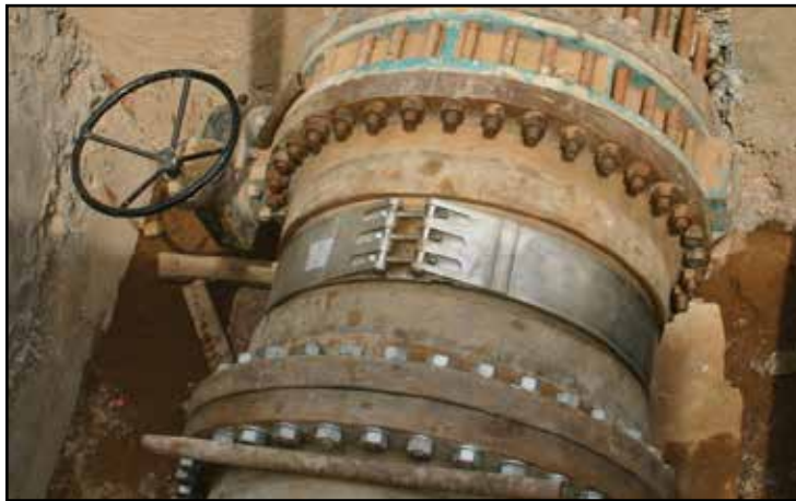
A 48 INCH ARMOR LINK™ CONNECTING TO A VALVE.
