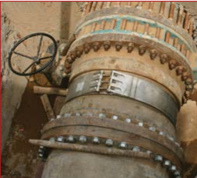
As the water pressure rises, the hydrostatic gasket seals tighter.
