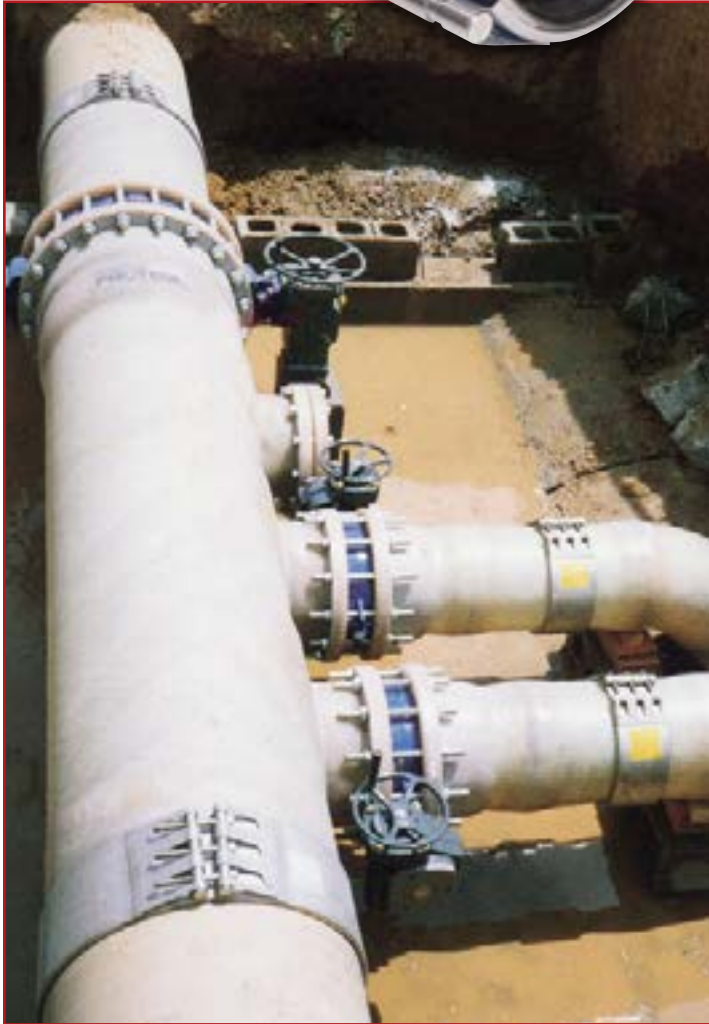
As the water pressure rises, the hydrostatic gasket seals tighter.
