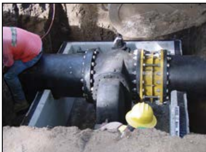
The Romac DJ400 combines a flanged spool piece with restraint tie-rods in one easy-to-use assembly.
