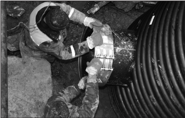
INSTALLING AN ARMOR LOCK™ ON A 16 INCH BRANCH.
