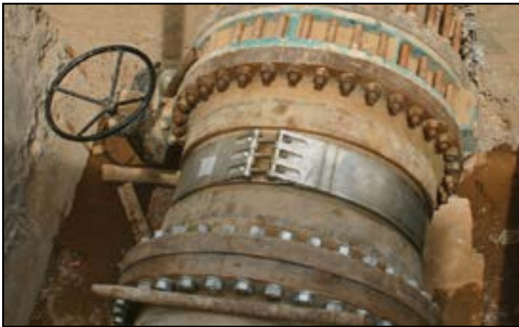
A 48 INCH ARMOR LINK™CONNECTING TO A VALVE.
