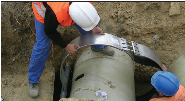
INSTALLING AN ARMOR SEAL™ ON A 24 INCH PVC PIPE.
